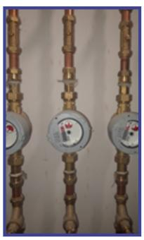
Stop valves allow you to shut off sections of the water system if there is a leak or if you need to change a washer or make alterations. It is a good idea to label your stop valves to remind yourself of their function. All stop valves should be kept easily accessible and operated at least once a year to keep them in good working order.
