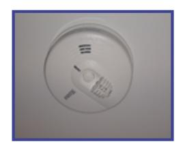
All of the apartments in the building have an open plan arrangement (i.e., no internal fire separation) which is classed as Category D LD1 detection. Therefore, all rooms except bathrooms are provided with a mains power smoke/heat detector alarm. All units within the flats are linked and will be activated if any of the detectors are initiated.
