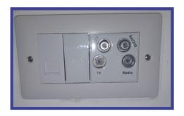
Communal Integrated Reception System (IRS) – this system includes a communal satellite dish, digital aerial and radio aerial and allows you to receive analogue, digital or satellite programming and FM and Digital Audio Broadcast (DAB) radio.
