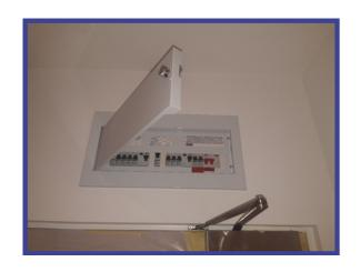
If a circuit is overloaded, a faulty piece of electrical equipment is used or there is damage to a cable, the circuit will switch off. If it is not known why there was a short circuit, switch the MCB back to on. If the switch will not stay on, you should establish if there is a faulty appliance by removing each one, one at a time, and switching the MCB back on after each.
